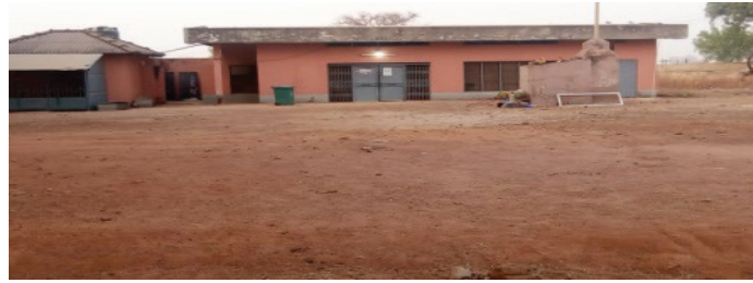
4.3 A picture of Bolgatanga mortuary where dead bodies have been kept Source: Researcher Constructs, 2020
