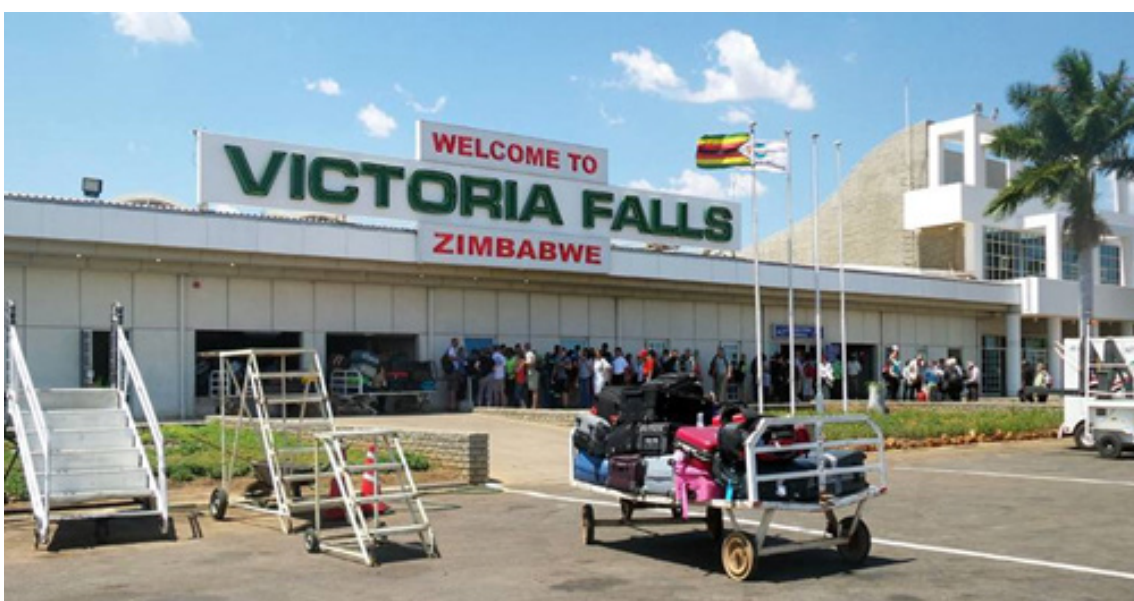
Figure 5: An image of the Victoria Falls Airport before its expansion
